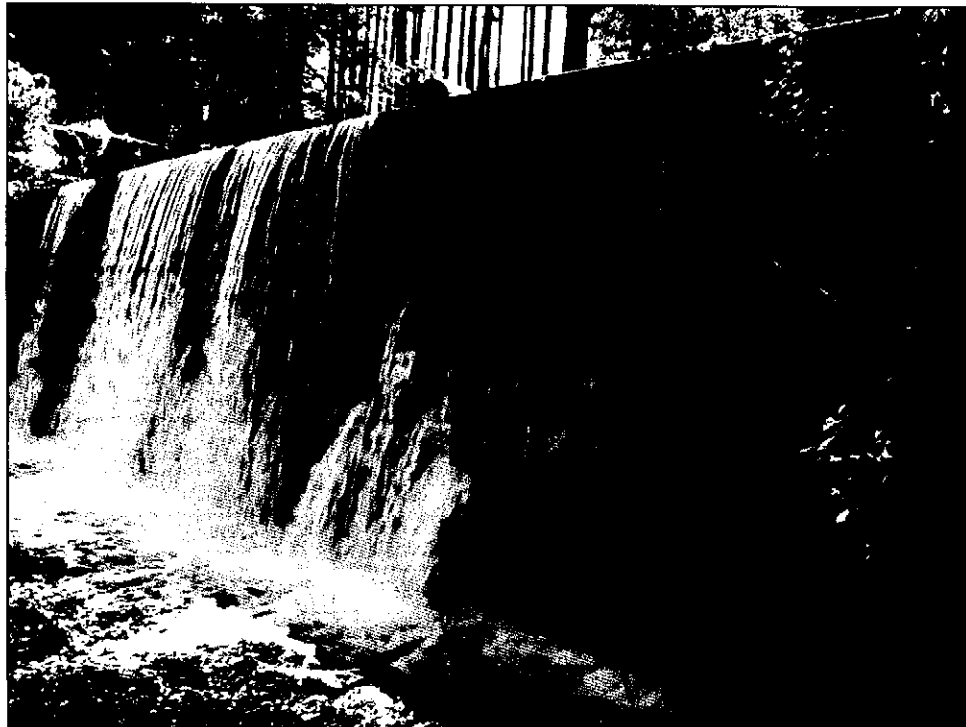
Photo 32: Water leaking through the auxiliary spillway downstream masonry face
