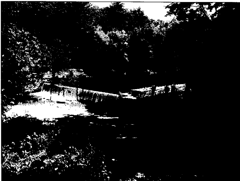
Photo 2: Overview of dam from downstream
